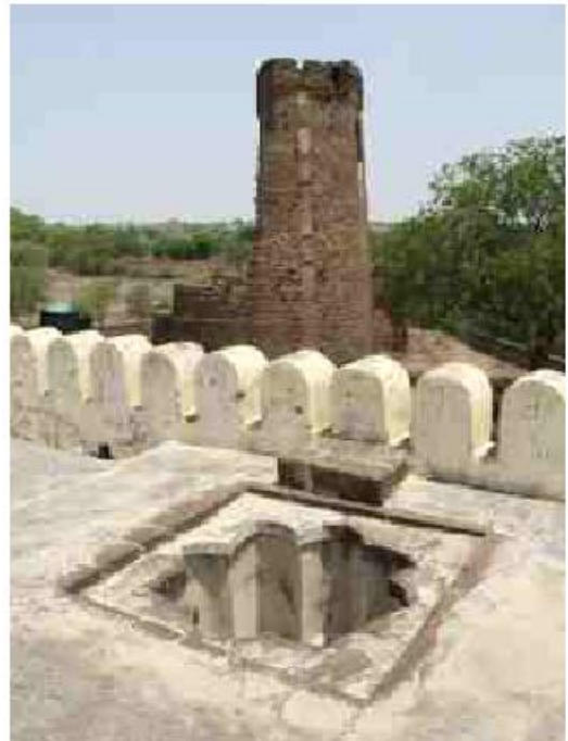
Open air bathing tub on the roof and over head tank tower - Kumatagi
