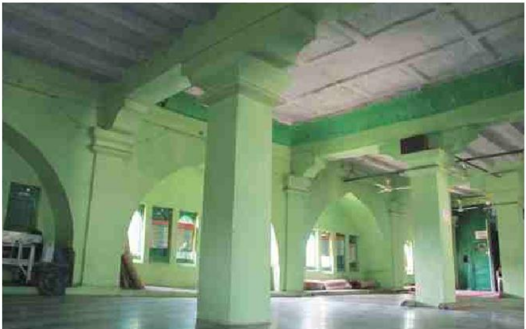
Arches, pillars & ventilation of western apartment
