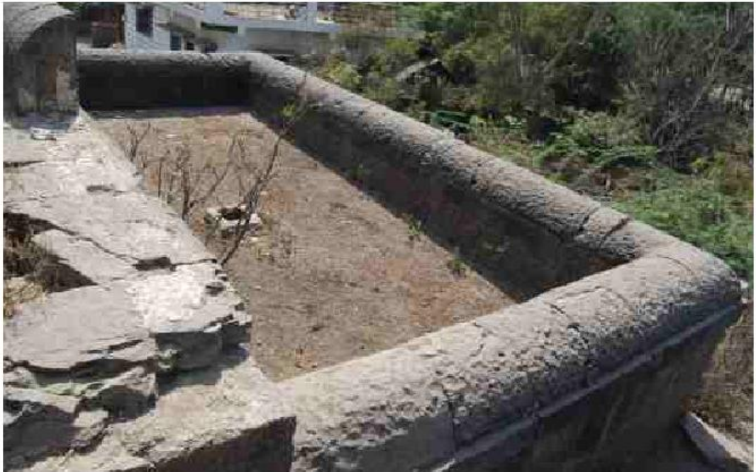
Roof Ventilator - Southern side
