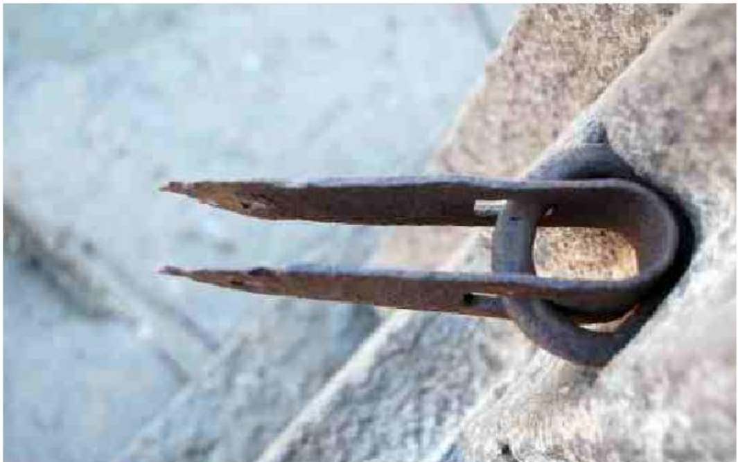
Iron Clamp for holding window panels of Minaret
