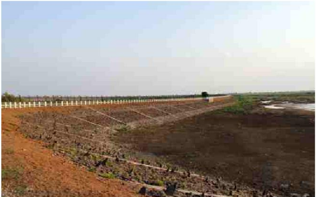
Renovated Jahan Begum Tank
