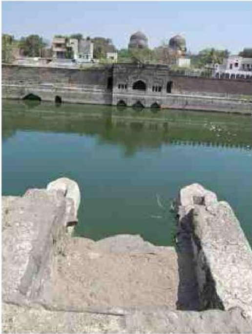
Western mot system
