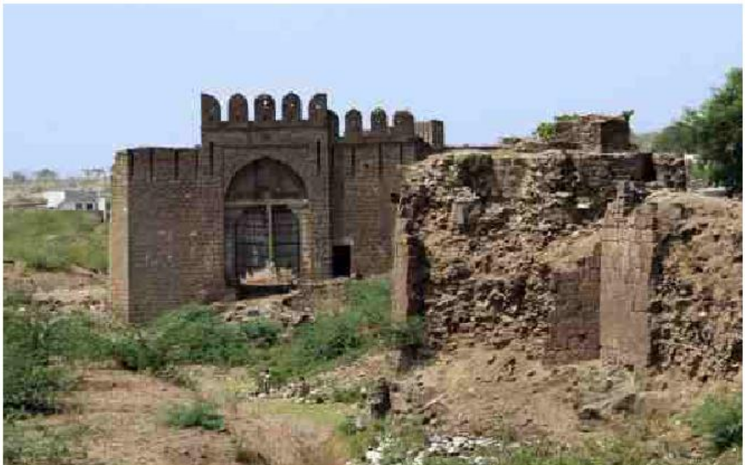
Allahpur Gate with broken fortwall
