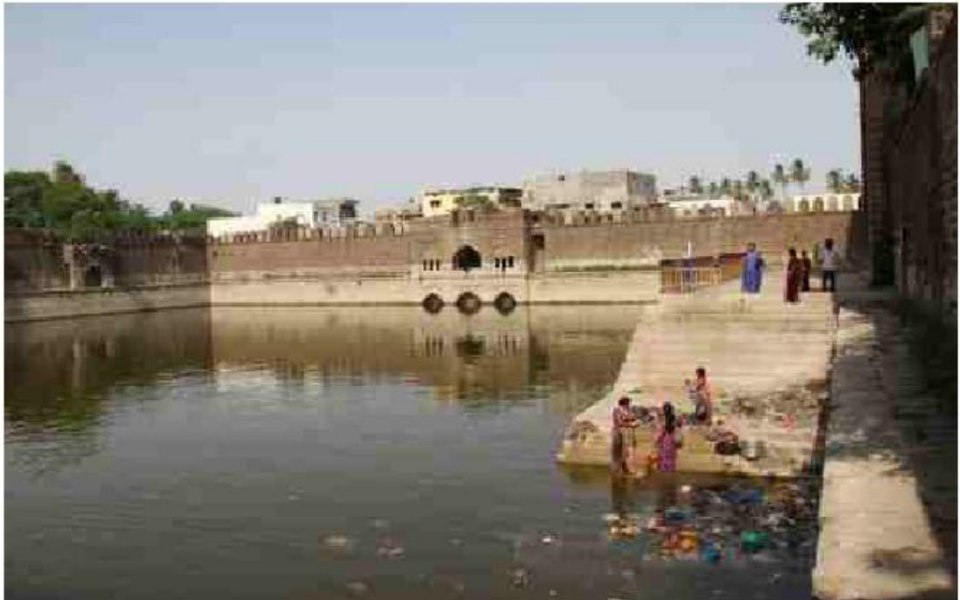
Pollution generated due to washing
